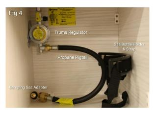
Most of our pod units are designed to run off Camping Gaz 904/7 cylinders. Inside the pod the cylinder is threaded onto the end of the Brass fitting with the red dial on top. The red dial is your Isolation knob, the gas supply should be turned off here when the hob isn't in use. There is a gas bottle strap within the pod's lower compartment, the bottle should be firmly strapped in place at all times. (4)
